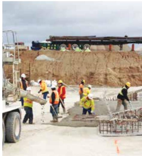
A concrete pour in action at the Trafalgar and Derry Road Feedermain and Reservoir project.
